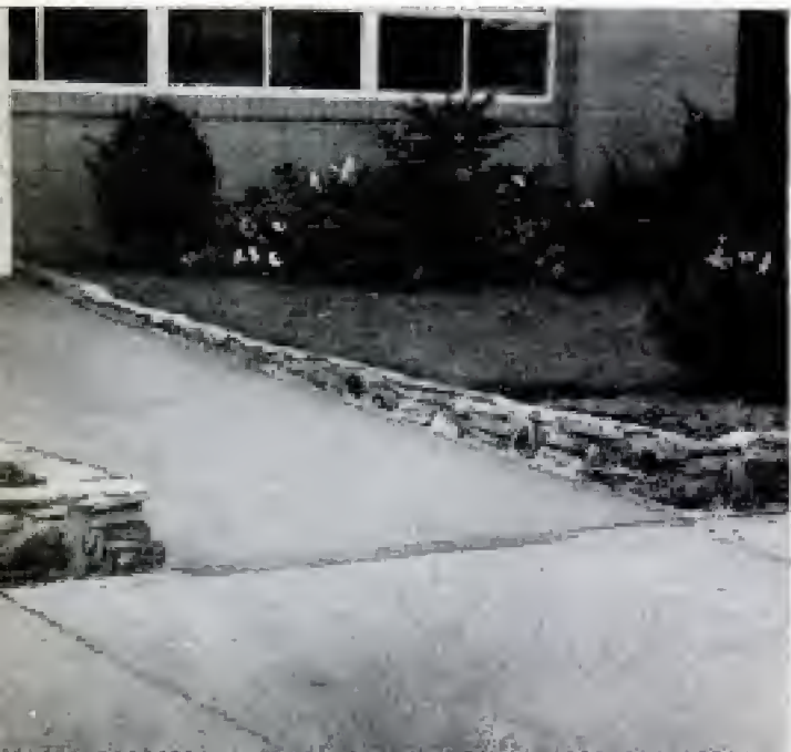
Wall just a few stones high keeps people off the grass and is a neat, attractive edging for sidewalk
